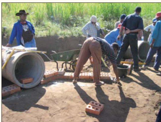
Construction of headwalls training at Chibini Road
