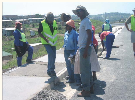
Contractors Being Mentored on How to Execute Steel Fixing and Concrete Jointing on P577 in KwaMashu
