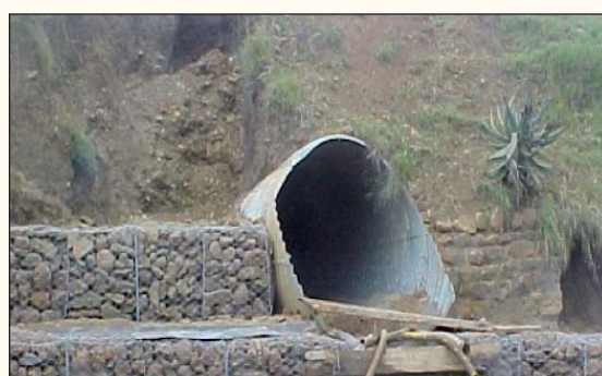
Repairs of Damaged Headwalls in Progress
