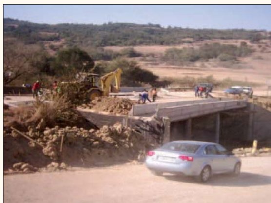
Droewig River Bridge No 2505 during Widening
