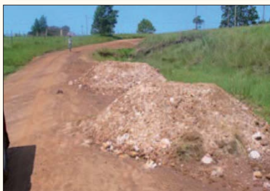
The 37km long P714 from Sibudo to Kingscliff being regravelled during the year
