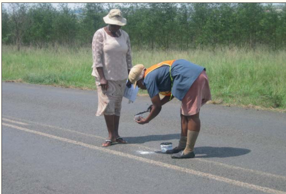
The CRDC Learner of Sinothemba Construction Being Mentored on the Installation of Road Studs on P154 in Wartburg
