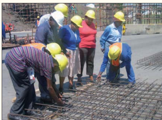
Contractors Being Mentored on How to Execute Steel Fixing and Concrete Jointing on P577 in KwaMashu
